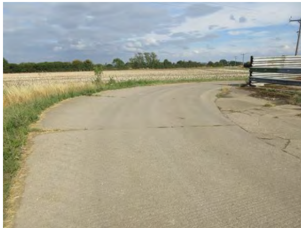
Photograph 11. Farm access track towards left hand turn. Load moves towards camera. Expected to be negotiable. Exact requirements to be confirmed once final loaded trailer arrangement known. Temporary plates on outside of the bend could improve turning radius or remove fence panel.
