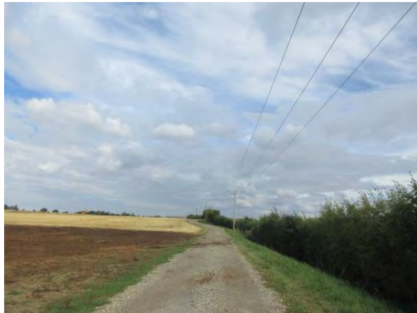
Photograph 17. Farm access track towards substation and transformer location. Load approaches camera. Negotiable with caution and confirmation of overhead clearances to power lines. Road width 3.4m.
