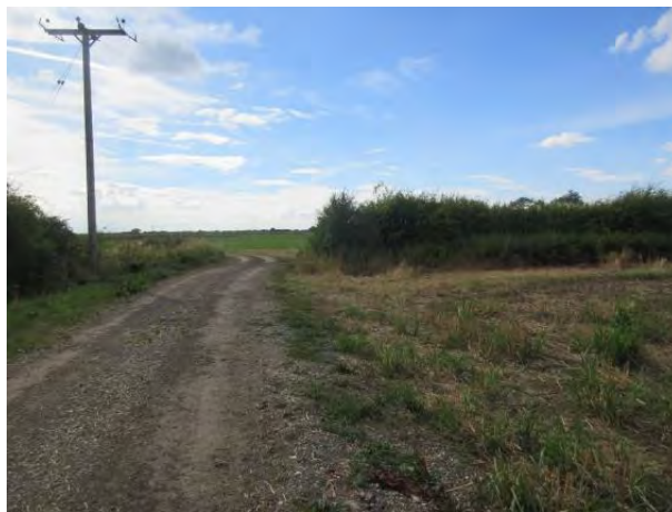
Photograph 20. Farm access track towards substation and transformer location which is on the right.. Negotiable with caution and confirmation of overhead clearances to power lines. New road construction to substation to be considerate of ALL loadings.
